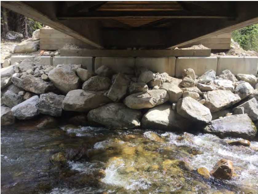
Left Bank Abutment when facing downstream
