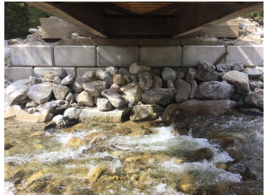
Right Bank Abutment when facing downstream
