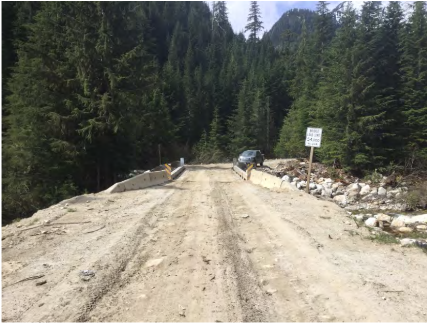
Approach from Left Bank when facing downstream
